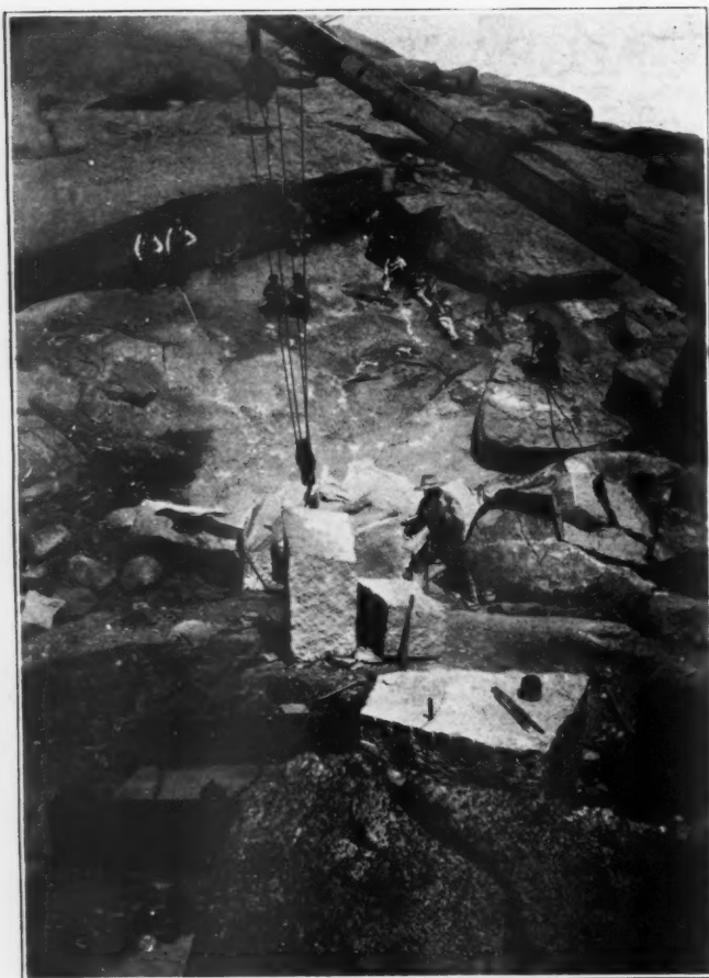
Getting Ready to Lift a Slab
